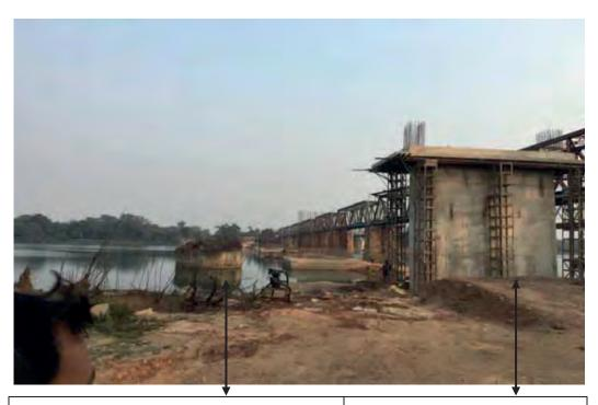
Figure 3.10: Abandoned constructed with Well foundation
