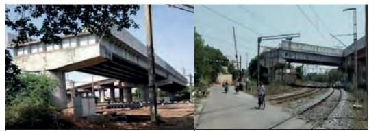
Figure 3.7: East Side (approach was Figure 3.8: West Side (Approach work completed but not connected to bridge yet to be taken up - May 2020) proper-May 2020)
