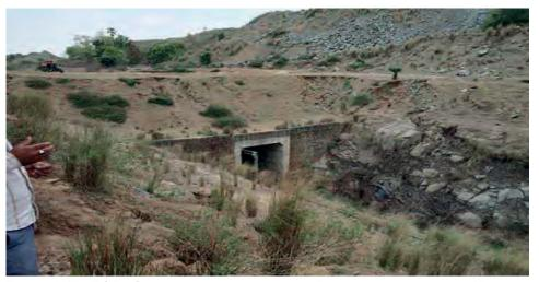
Figure 2.10: ECR: Overpass constructed over Railway track between Khurhagora and Kathautia stations for safe passage of elephants
