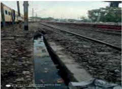
Figure 4.1: Sewage of Platform No.03/04 blocked with Ballast at Gaya (ECR).
